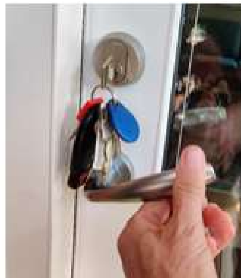
ALWAYS ENGAGE MULTI-POINT HARDWARE BY RAISING THE HANDLE UP BEFORE LOCKING THE DOOR
