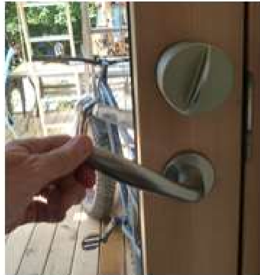
HANDLE UP TO ENGAGE MULTI-POINT HARDWARE
