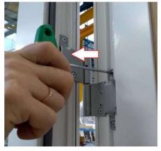
b) Next, using the 3mm Allen key, rotate the set screws (shown with the letter B above), ensuring that the adjustments are done evenly so the door is not twisted.
