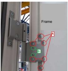
The adjustable hinges include a vertical adjustment screw (+/- 2mm) as shown in the left picture above. The hinges can be also adjusted in a horizontal direction using the screws marked with the letter B in the picture above, on the right.
