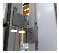
c) Using a Torx 20 screwdriver, tighten all previously loosened screws (shown with the letter A above).
